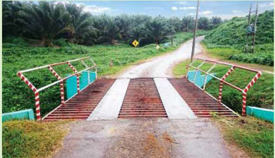
Estate access roads
